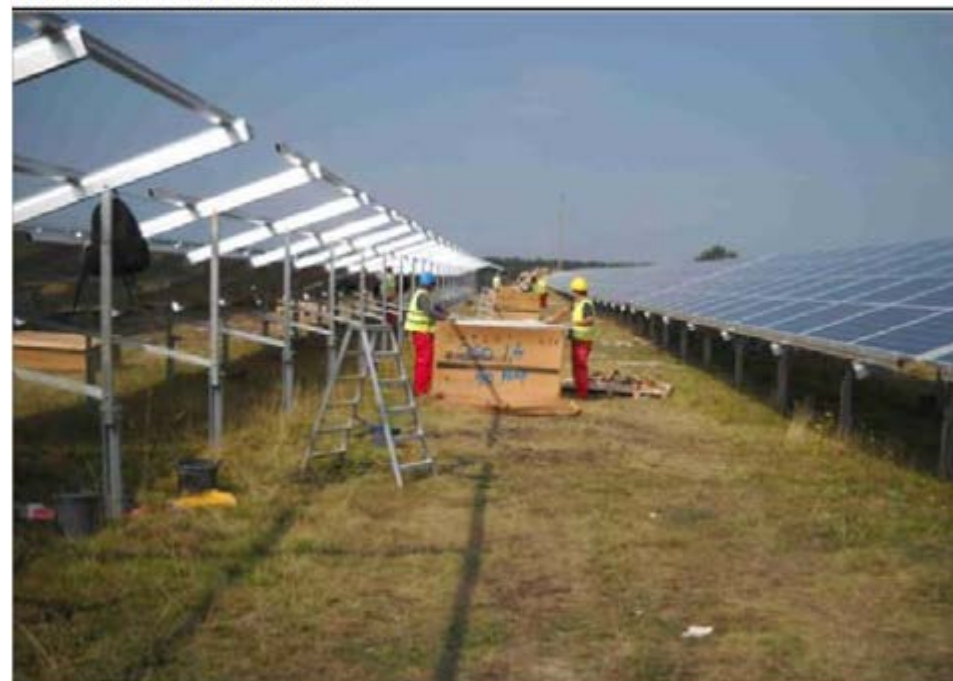
Modules installation
