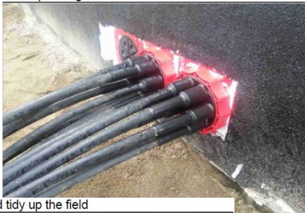
Waterproofing the cable after connection
