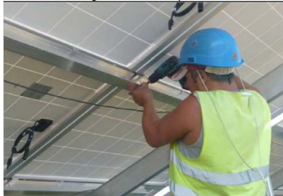
Installation of diagonal and lateral protection for modules
