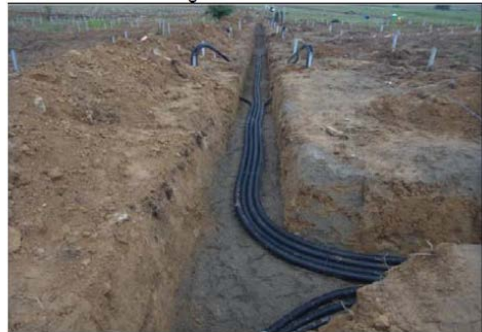
Trenches and Ducting
